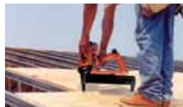
Plywood attachment—using TrakFast plywood to steel pin
