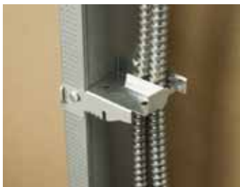
Metal Stud with MC/AC Cable
