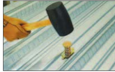
Metal-Deck Insert Installation Sequence
