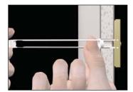
Hold ends of straps together between thumb & forefinger and pull toward you until channel rests behnd wall. Ratchet cap along straps with other hand until flange of cap is flush with wall.
